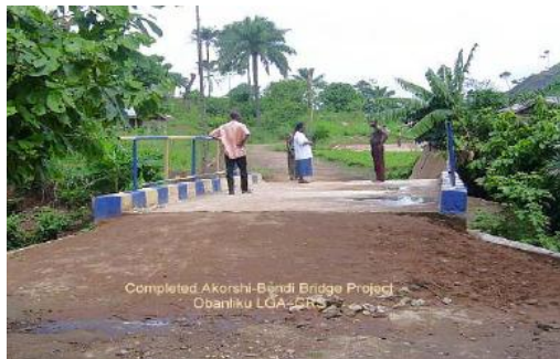
Akorshi – Bendi Bridge – Cross River
