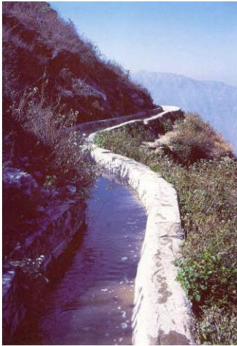
Rehabilitated irrigation canal - Nepal
