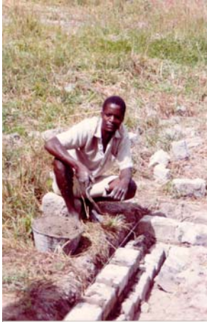
House construction using burnt bricks
