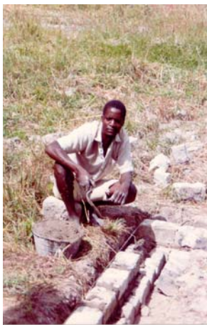
House construction using burnt bricks
